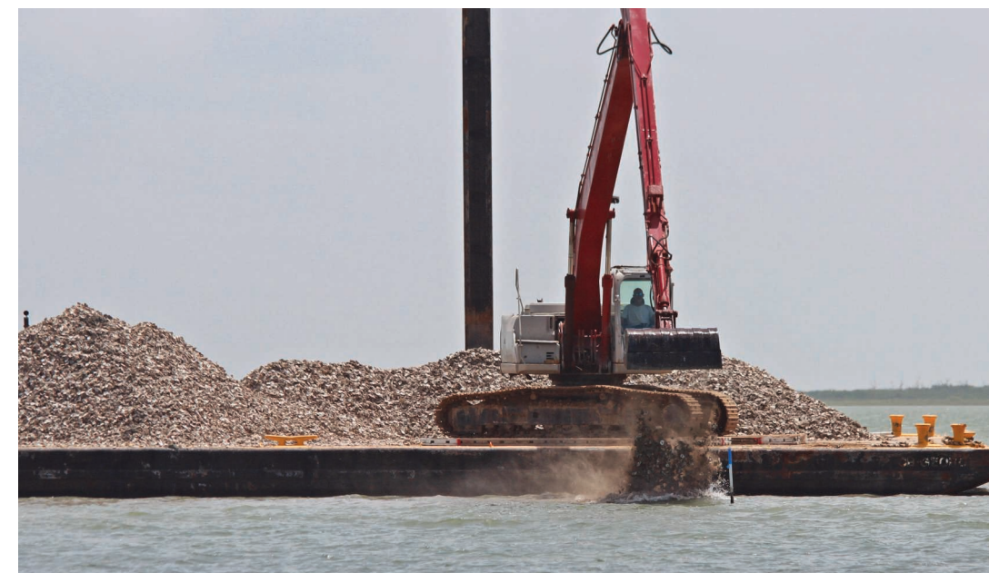
Derrick construction operators place shell in new St. Charles Bay Reef
