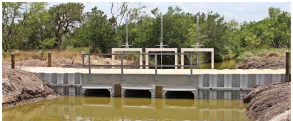
Water control station for the Nueces Bay Delta.
