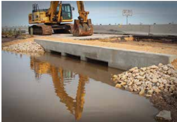
New culverts in marsh restoration project at Egery Flats in Upper Copano Bay.
