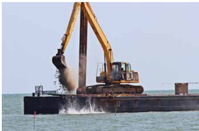
Placing shell on new reef site in St. Charles Bay
