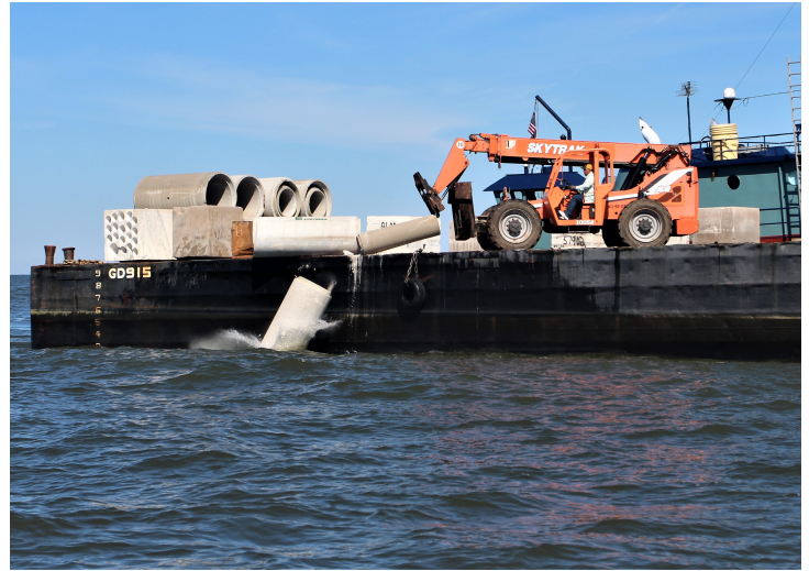
Nearshore reefing sites are composed of many materials such as these used at Sabine HI20 site.
