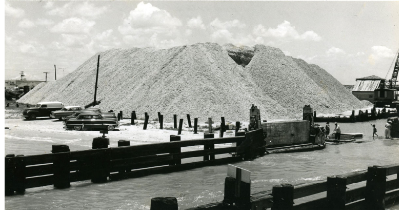
Stockpile of dredged oyster shells at Nueces Bay containing 50,000 cubic yards of shells. Corpus Christi Caller Times, July 16, 1955.
