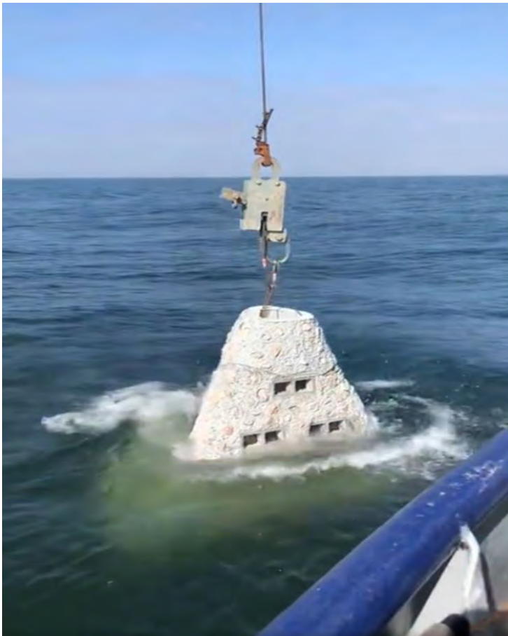
Big Man's and Kate's Reefs: One of the pyramids designed by Atlantis Marine Habitats being lowered to the bottom. Photo Courtesy of Laredo Construction
